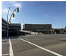
San Bruno BART Station Area
