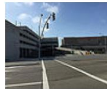
San Bruno BART Station Area
