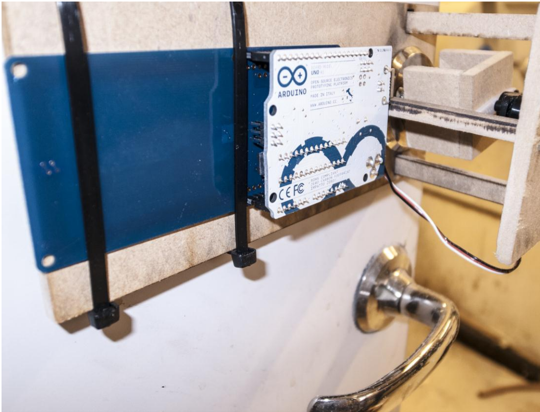
Figure 6.8: The final door lock in place
