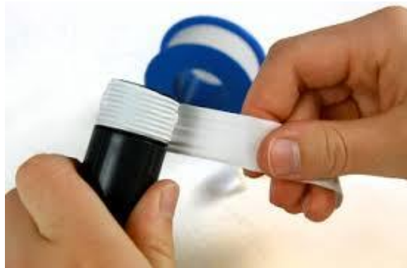
Securing the connection between water flow meter and BNC pipe connector using thread seal
